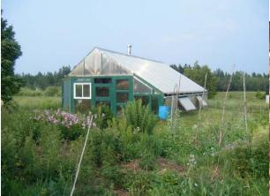
The 20 by 40 foot passive solar greenhouse is built of hemlock wood sitting on a fourfoot deep cement foundation. The south facing roof (on a 35 degree angle), and knee wall is made of a three-layer sheet of polycarbonate purchased at Halifax Seed.
